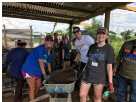
A Project Hope mission team works on a construction program. (RNS
