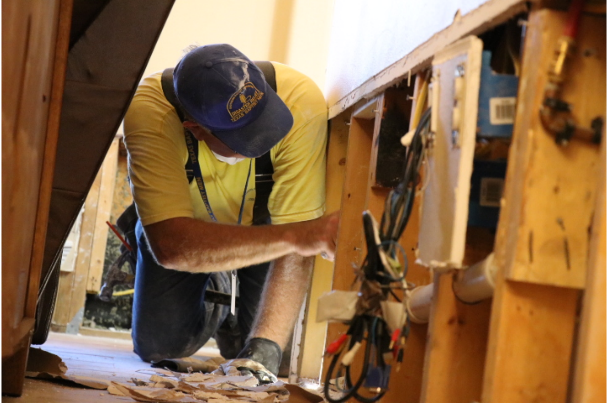
Jerry Hall from Ellis Baptist Association removes damaged drywall from a flood-affected home in Weslaco. (Photo / Rand Jenkins / TBM)
