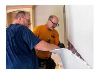
TBM disaster relief volunteers remove water-damaged drywall from the home of Bruce and Renee Smith in Mauriceville. (TBM Photo /
