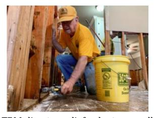
TBM disaster relief volunteers pull remaining nails after removing damaged drywall from the home of
