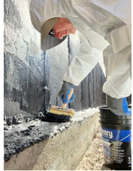
Wayne Pritchard, TBM Builders leader, applies sealant to the edge of the parsonage basement. (Photo / Ferrell Foster)
