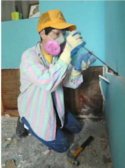
Mary Bess Jackson removes damaged drywall in an El Paso home.
