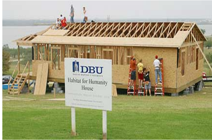
DBU Freshman Kendra Roberts puts the finishing touches on a Habitat home in Dallas. (Photo by Chris Hendricks)
