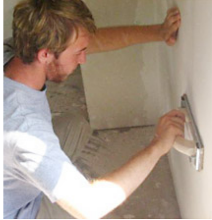
Josh Rhodes, a transfer student at HPU, helps with the dry walling in a home that was recently built in Cross Plains.
