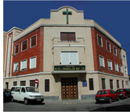
Texas Baptists built this church in Spain about 40 years ago.
